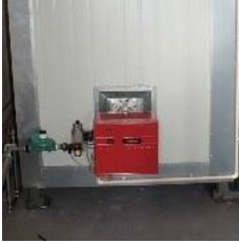
Figure 11: Heating System Housing for Colo
